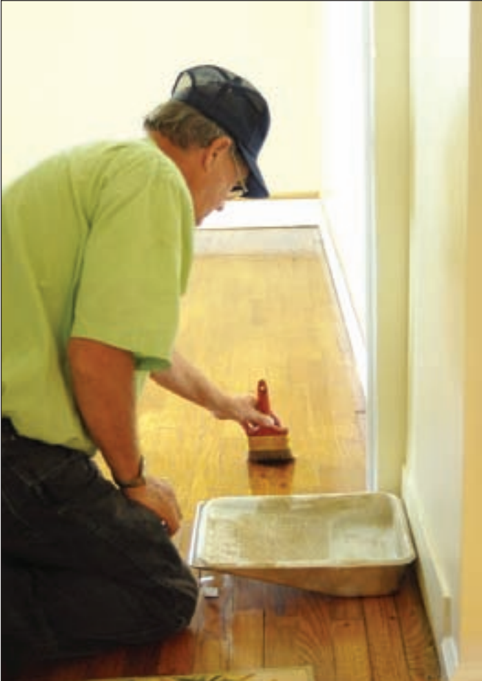
Donald Winders applies varnish to the floor of one of the home's two bedrooms.
